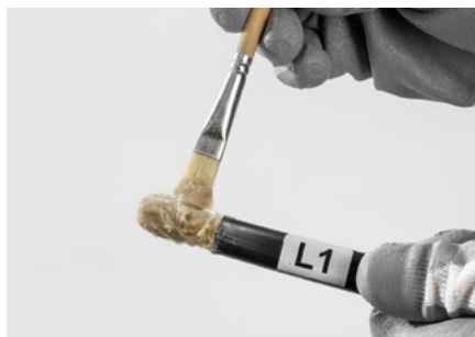
Cover the conductor all around with neutral grease.
