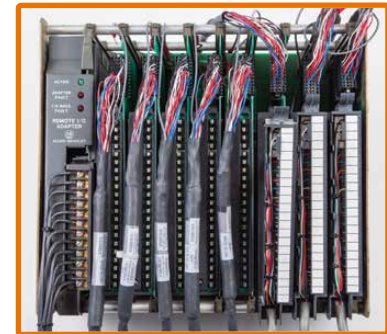
Reattach existing Field Wiring adaptors
