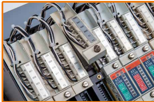
Reattach existing Field Wiring adaptors
