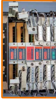
Remove existing Field Wiring adaptors
