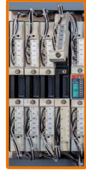
Replace controller card with Weidmuller adaptor card
